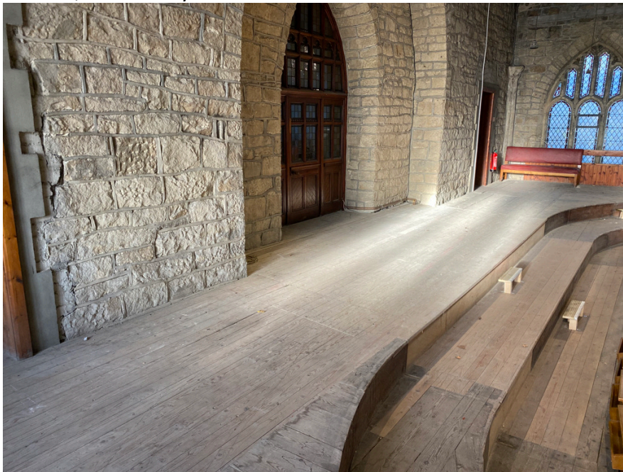
Photo 3, The Gallery area at the west end of the church where the chairs will be placed
