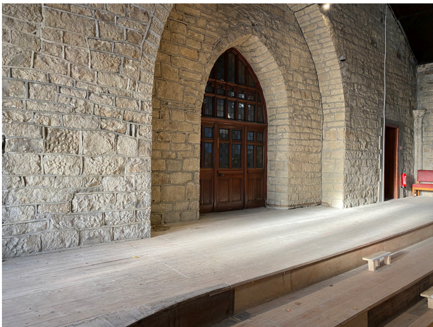
Photo 4 view of area where the chairs will be located
